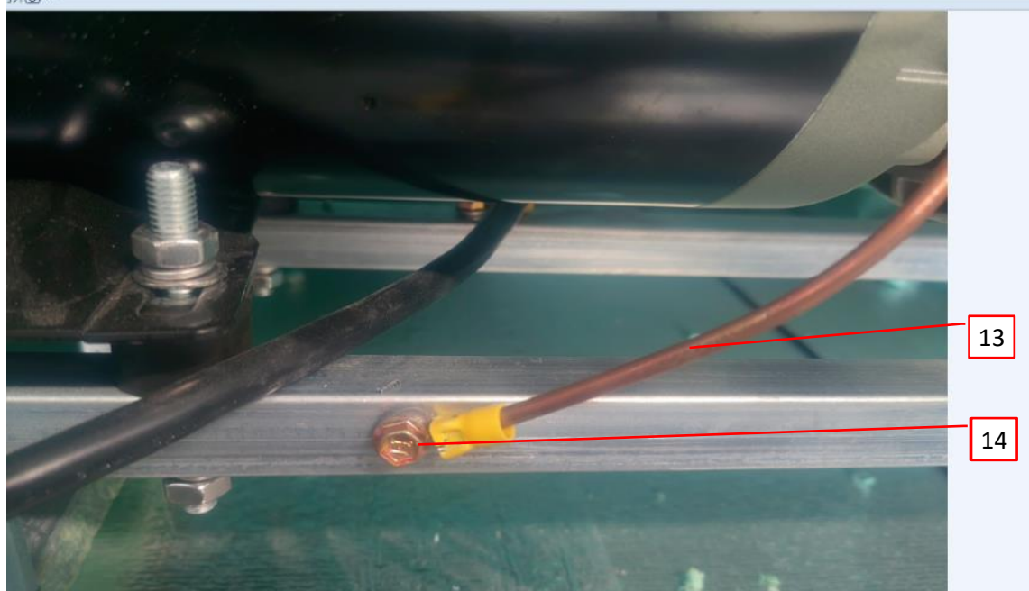
Photo 52 - Grounding Bonding each pump with bonding conductor.
