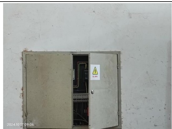
NC-PA7.13-The outer protective covers were not locked and inner protective covers were lost 1
