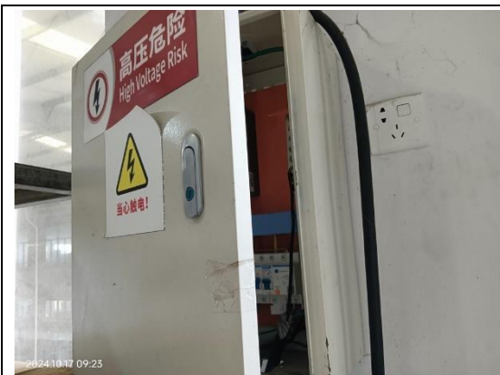
NC-PA7.13-The outer protective covers were not locked and inner protective covers were lost 2
